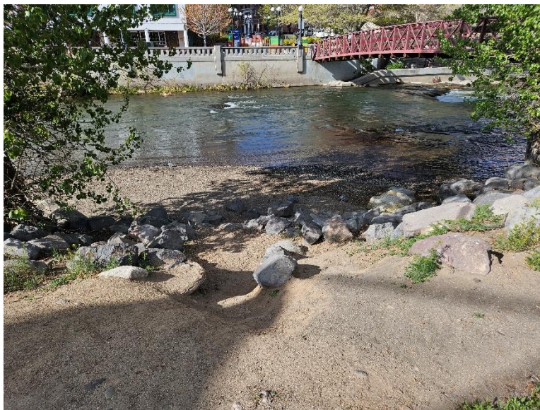
Eroded path down to pool 3
