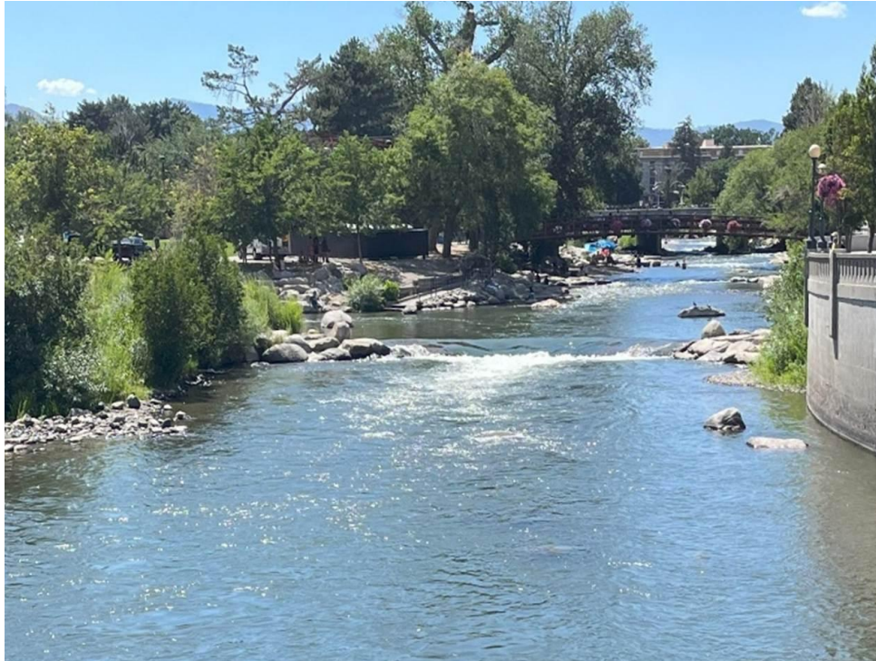
Current Conditions: Remaining tailwater control boulders visible at the left flood wall and right bank, but thalweg is impacted such that grade control is no longer provided.
