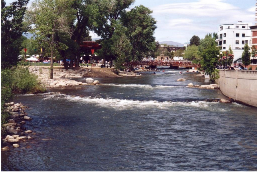
Original Design: Tailwater control structure in foreground, drop structure 5 in background.
