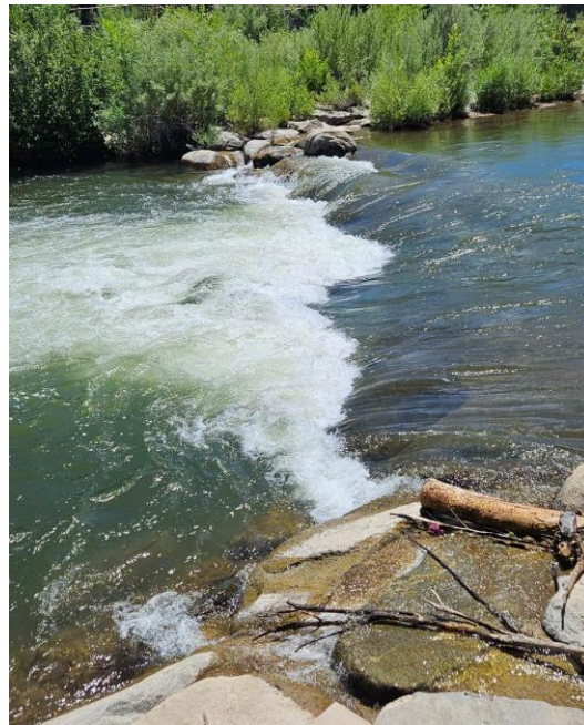
Current Conditions: Recirculating, powerful "plunging conditions" hydraulic jump due to dropping off the end of the structure and higher than designed head differential
