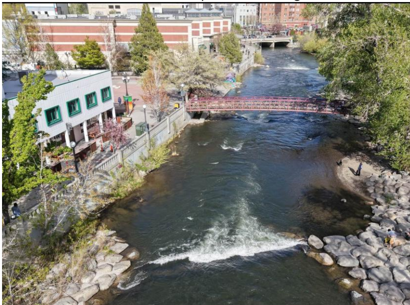
Current Conditions: Accumulated sediment, especially evident at right bank. Drop Structure 4 is drowned out due to downstream deposition.
