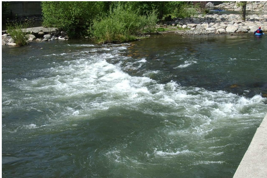
Original Design: Tailwater control structure maintaining grade upstream (right)
