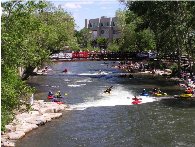
Original design: Deep water downstream of Drop Structure 3, pronounced Drop Structure 4 is visible downstream of pedestrian bridge.
